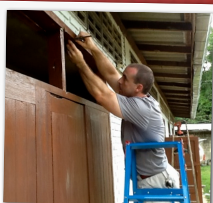
INSTALLING NEW WINDOWS AT YOUTH HOSTEL
